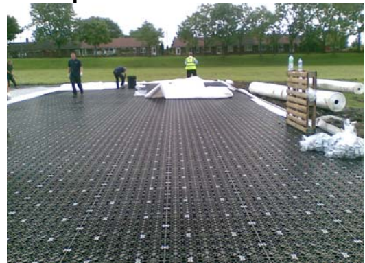
SudsSports in Pitch Construction
