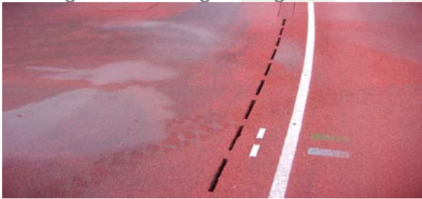
Clearing out & Cleaning Drainage Channels
