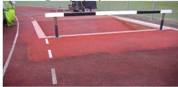
Refurbishing Steeple Jump Pits
