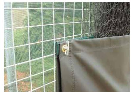
Net storage pouch fixing detail
